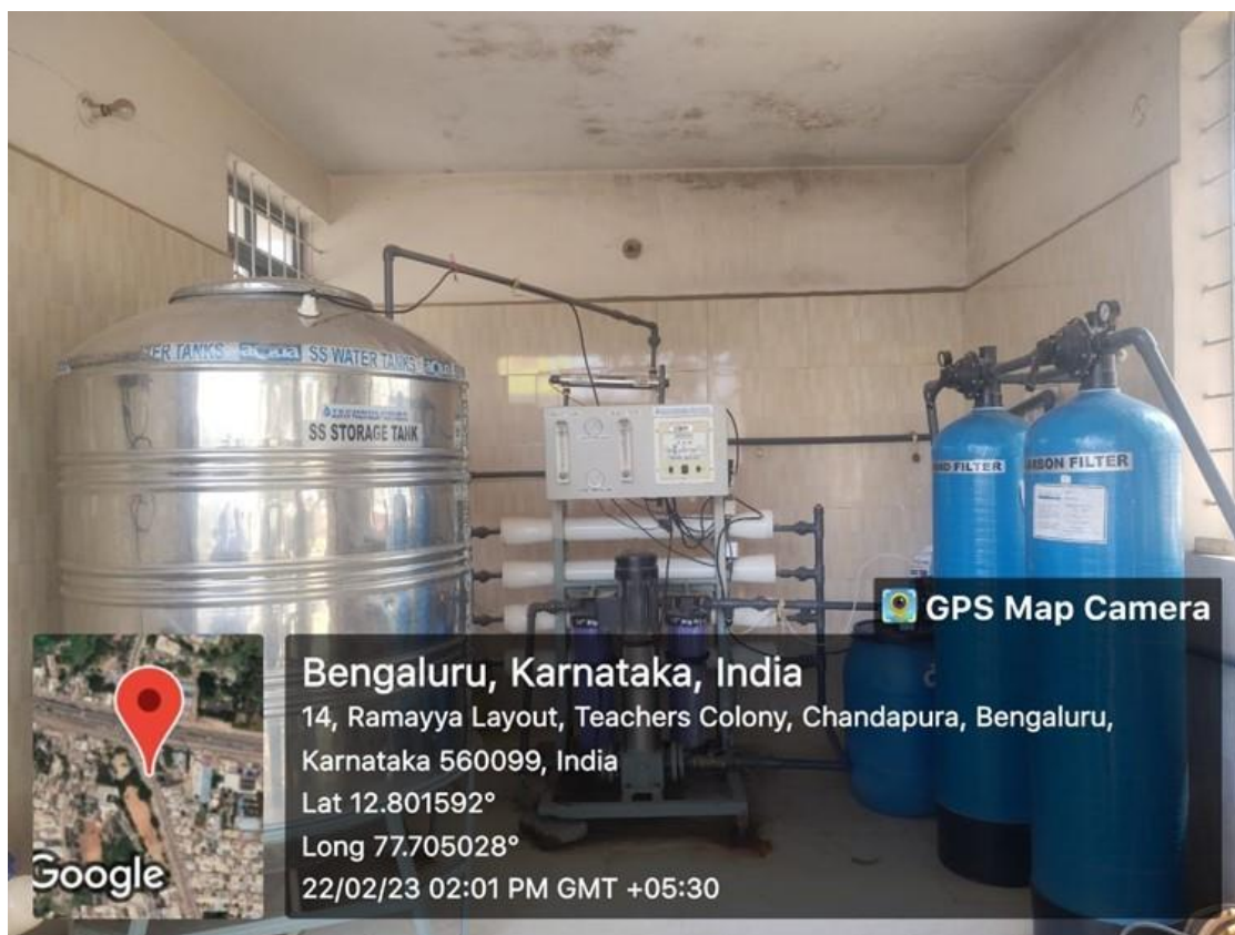
Figure 4-7: RO plant installed in the campus
