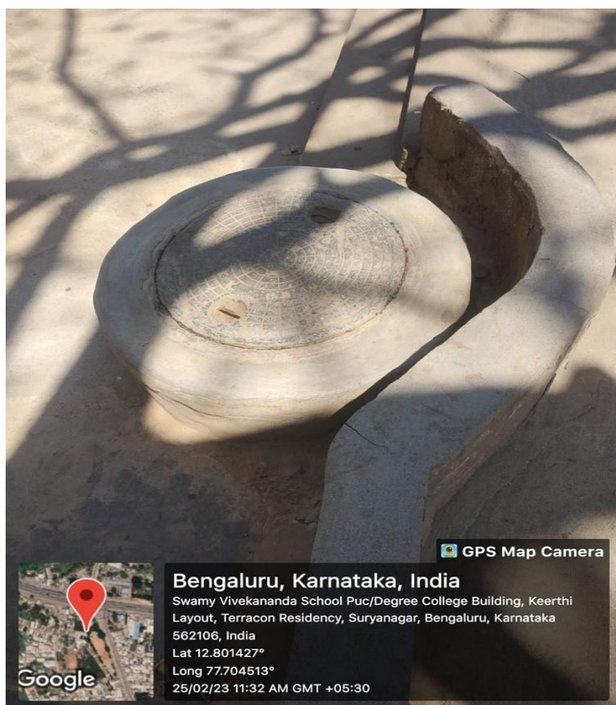
Figure 4-13: Waste water chamber
