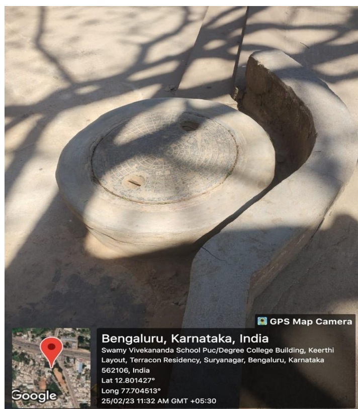
Figure 6-2: Waste water chamber
