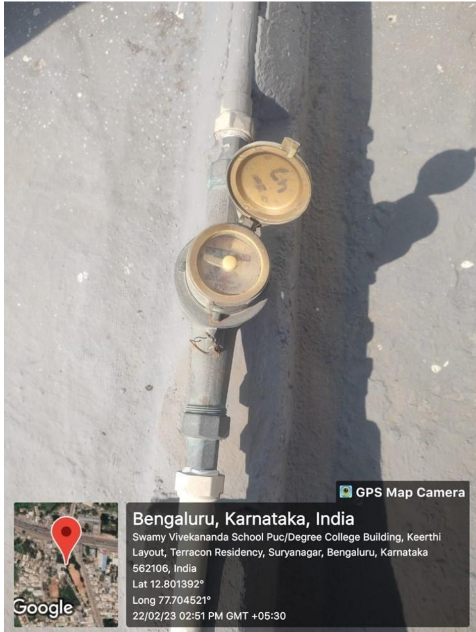
Figure 4-15: Water flow meter installed in the terrace
